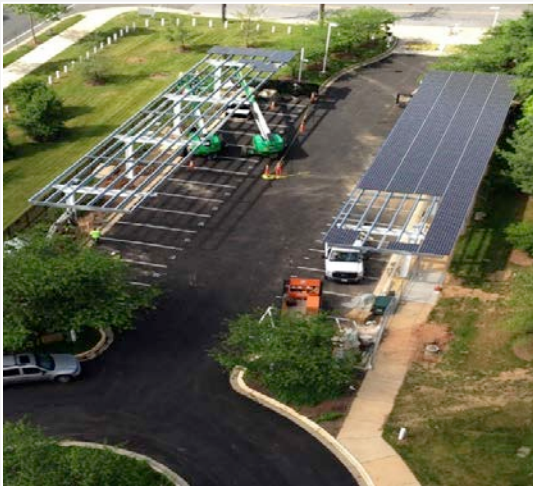
New Carrollton, MD Federal Building ESPC project : solar carport, geothermal, fields, chiller plant upgrade
